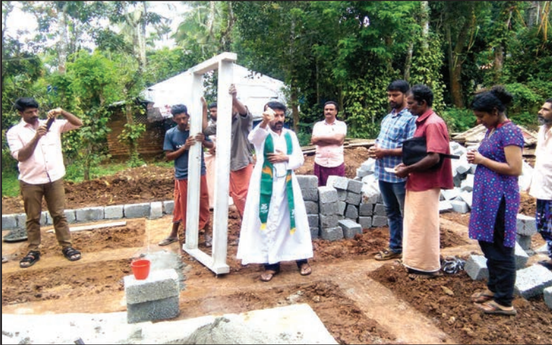
House Project in progress @ Pious Nagar Wayanad
